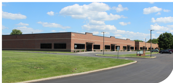
New facility in Norriton Business Campus
